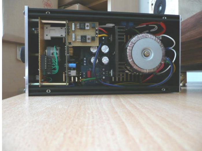
Photo 2: Physical arrangement of the different blocks in the cabinet
